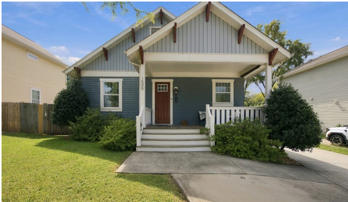
Craftsman brackets, board and batten gables, and a covered front porch on Norris Ave
