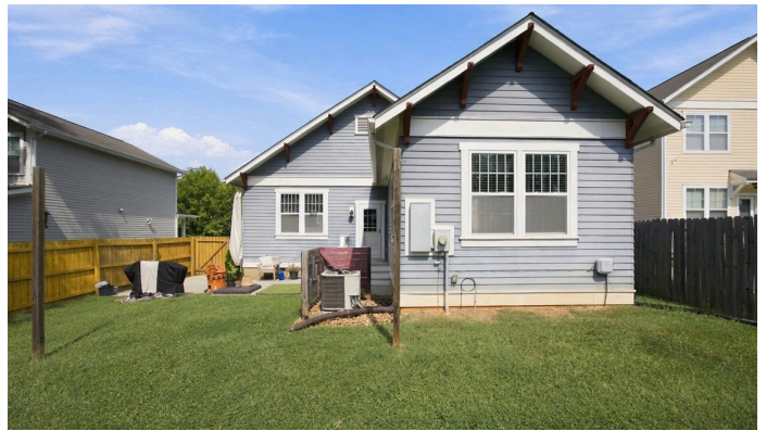
The rear of the home, fiber cement and wood siding, with the heat pump and utilities tucked to one side
